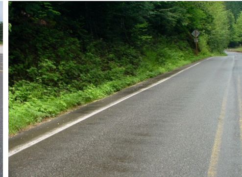
Examples of deficient Paint Stripe
