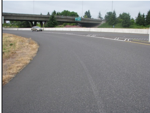
Examples of deficient Paint Stripe
