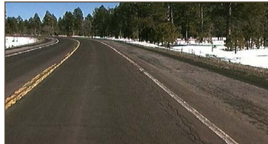
LOS B: This pavement is in good condition with good ride quality.
