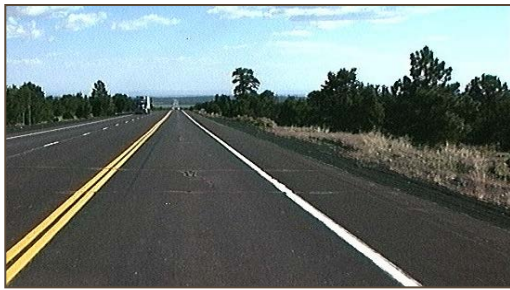
LOS A: This pavement is in very good to perfect condition.
