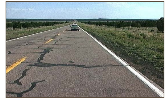
LOS C: This pavement is in fair condition with fair ride quality.
