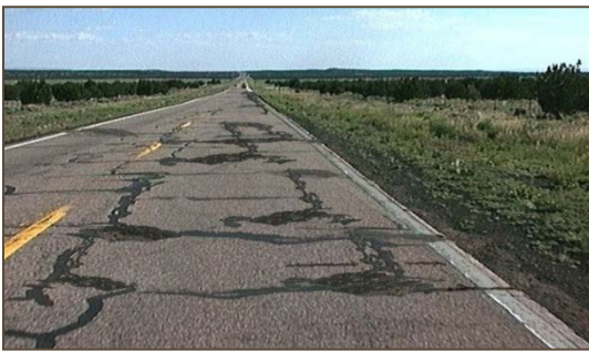
LOS D: This pavement is in poor condition with poor ride quality.
