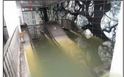
Figure T-03: Escalators under water at the South Ferry subway station. (MTA, 2012)
